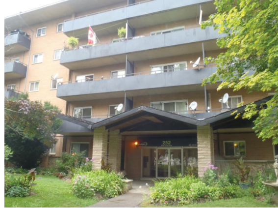
252 King Street East – Bowmanville, ON
