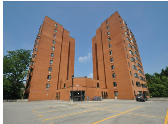
545-565 Belmont Avenue – Kitchener, ON
