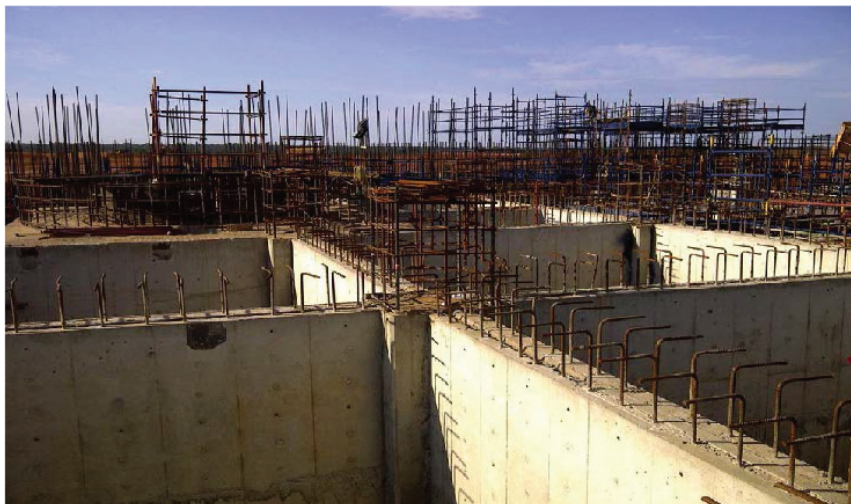
Copper smelter under construction
