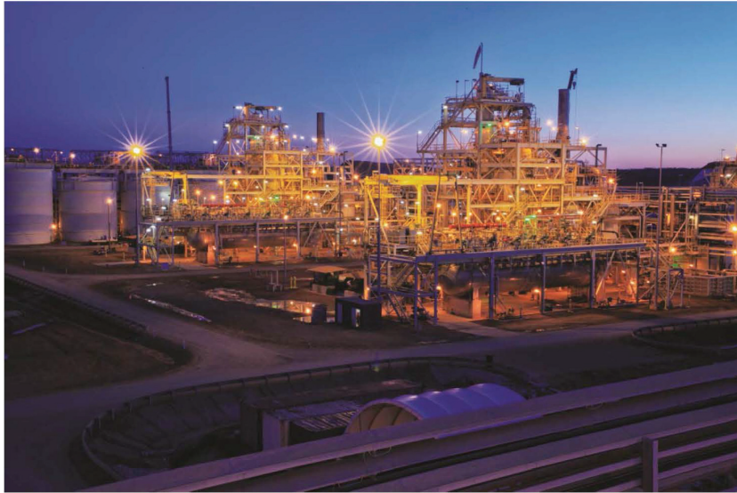
Ravensthorpe Mine processing plant
