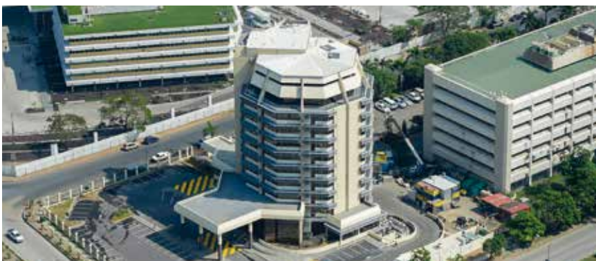
Manasupe Haus, one of two NITCS projects completed in 2015, was officially handed over to the Department of Prime Minister and National Executive Council in January 2016.
