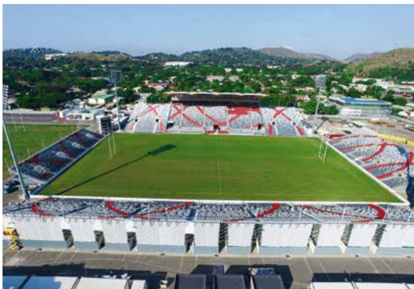
The National Football Stadium, one of nine infrastructure projects managed and delivered by Oil Search on behalf of the PNG Government in 2015, hosted its first game in February 2016.
