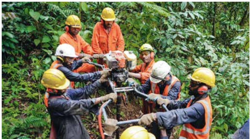
Seismic acquisition in the PNG Highlands.
